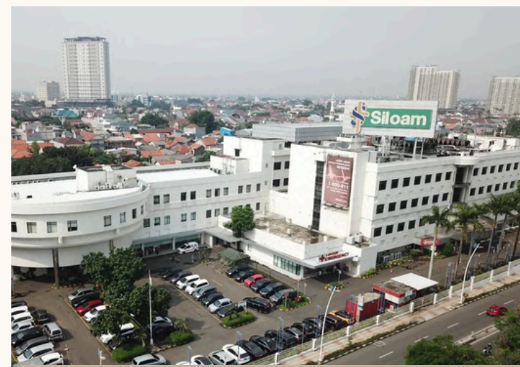
SILOAM HOSPITALS KEBON JERUK
